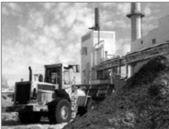
A power plant in the US, which produces electricity through gasification of wood chips
